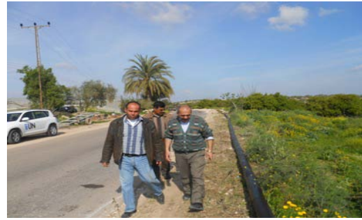
Checking pipes specifications in the field and supervising the installation / Tulkarem
