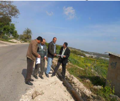
Installing the main irrigation network
