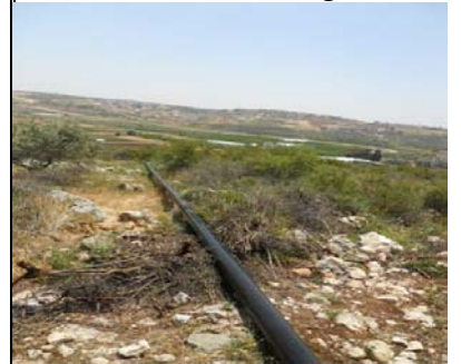
Installing the main irrigation network
