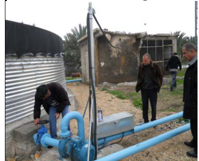
Installing the main irrigation network
