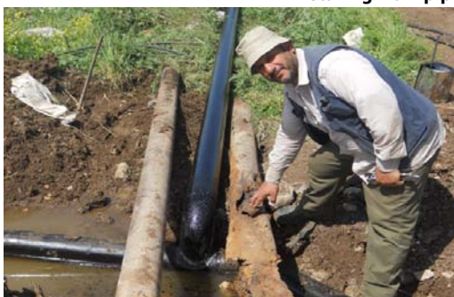
Rehabilitation of irrigation system New pipes Vs. old pipes / Qalqiliyah
