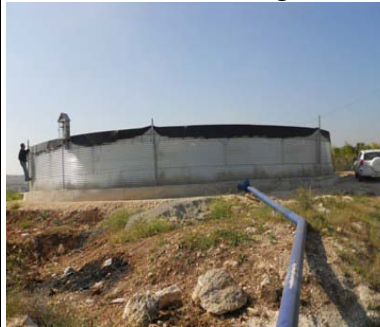
Installing the main irrigation network
