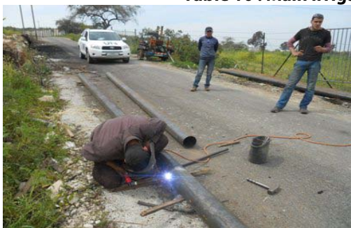
Installing main pipelines / Qalqiliyah
