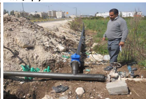
Upgrading of the irrigation system to serve new areas / Tulkarem
